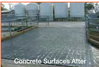
Cattle Underpass After
